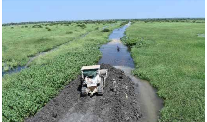
Rehab of Main Supply Route
